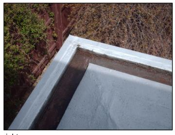
Standing water / ponding water was observed in the gutter at the left side of the back bump out. This suggests that the gutters are no longer pitched consistently towards the downspouts. This can accelerate deterioration of the gutters. This condition is illustrated in the accompanying photo right.
