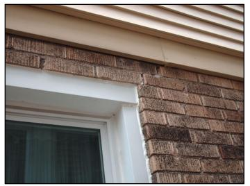
16. Loose and missing mortar was observed in the brick window sill to the first floor window on the left side.
