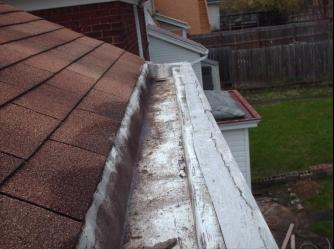
Surface rusting was observed at the upper level front and rear gutters. Painting maintenance is recommended. This condition is illustrated in the accompanying photos.
