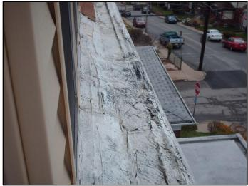
The front porch and back addition had been coated in aluminized roof paint. There were areas at the back addition that the paint was beginning to bubble and peel away. It is recommended that these areas be repainted to prevent excess rusting and deterioration of the metal roofing and box gutter. This condition is illustrated in the accompanying photo above left.
