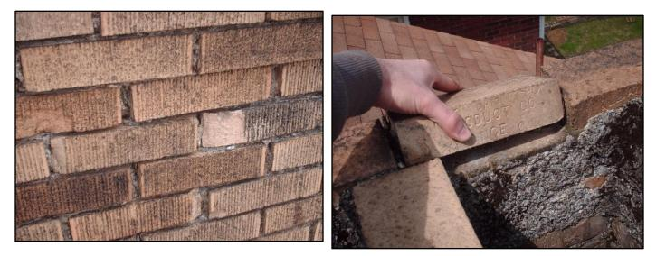
Loose and missing mortar was observed at the back left side chimney. There was no cement crown at the top of the chimney. There was loose brick observed at this chimney as well. This condition is illustrated in the accompanying photos above. 26. The original box gutters are still in use at the main roof and front porch and rear addition.
