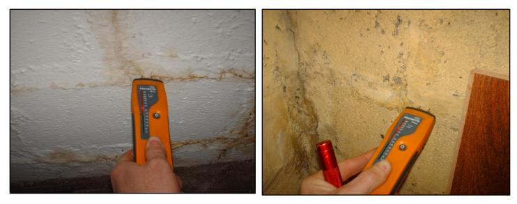
28. Staining, efflorescence and signs of past water penetration were observed on the foundation walls at the front right corner of the basement. When checked with an electronic moisture meter, some of these areas were wet or damp at the time of the inspection (35% - 45% moisture). This condition is illustrated in the accompanying photos above.
