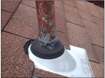
caulking to reseal the plumbing vent flashing at the back side of the roof. This condition is illustrated in the accompanying photo right. It is recommended to monitor this area for signs of future leakage. Resealing or re-caulking this joint may be necessary.
