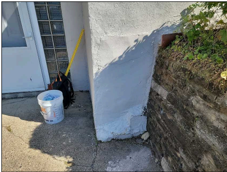
Cracks to the parge coat at the front foundation wall
