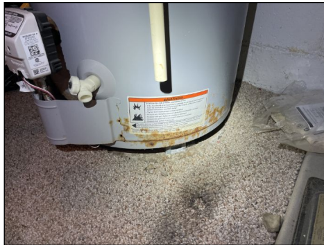
Rust on the bottom of the water heater
