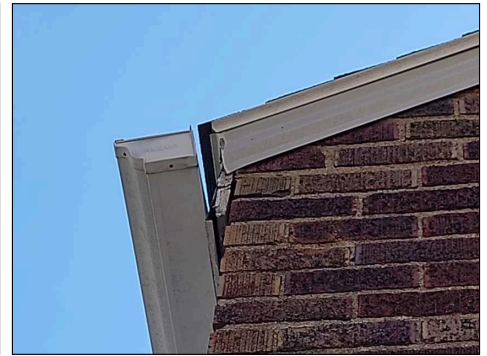
Gutter pulling away from fascia
