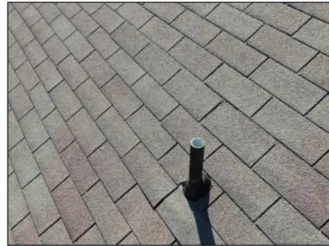
Shingles installed over bottom apron of plumbing vent flashing
