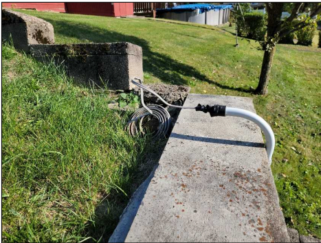
An exposed wire was observed at the back exterior
