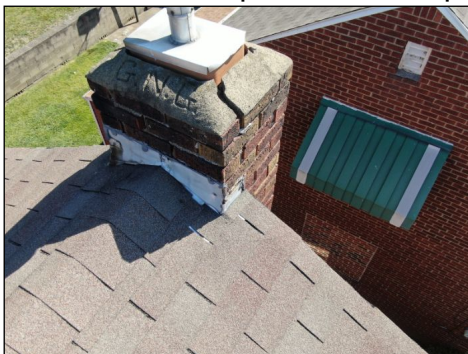
Cracked chimney crown
