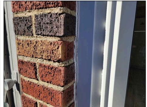
Dried and cracked caulking around windows and doors
