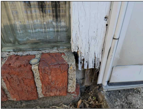
Rotted wood observed at the front basement door
