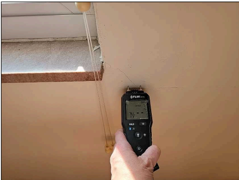
Repaired areas and cracks were observed around windows
