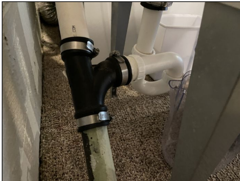
S-trap below laundry tub
