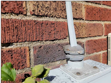
Duct seal at the top of the electric meter socket deteriorated
