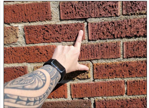
Step crack observed under the front right window.
