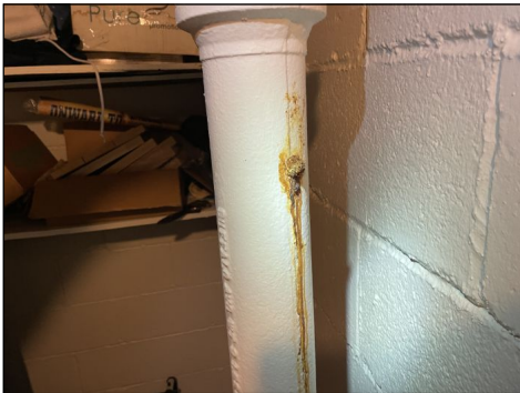
Rust blisters on drain stack
