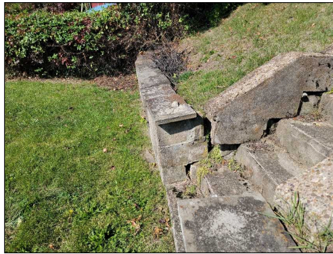
Retaining wall movement near back steps
