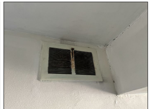
Open vent in left room of basement that may need to be sealed off for future garage
