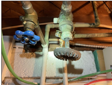
Corroded valves that may not function properly
