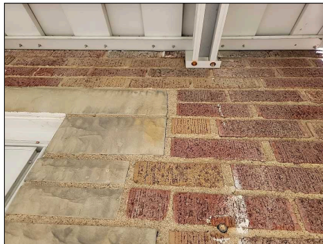
Hairline masonry cracks around some of the doors and windows
