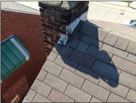
Chimney flashing needs to be resealed
