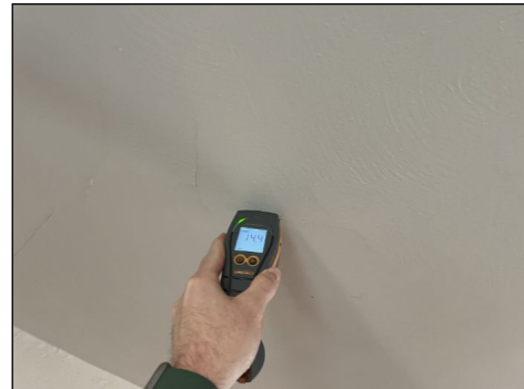
Stain and cracks to living room ceiling from bathroom leak
