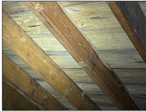
Staining on roof nails to roof deck in attic
