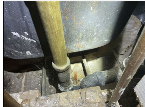
Leakage from tub to second floor bathroom
