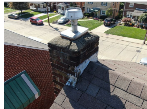
Loose mortar to the chimney
