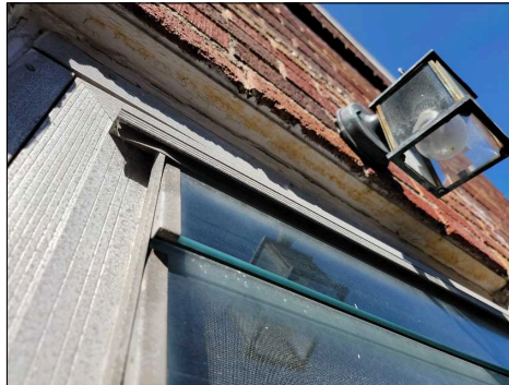
Rust on the steel lintel above the door
