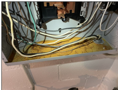
Rust at bottom of main panel
