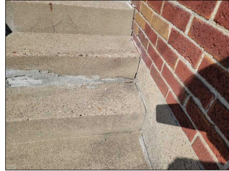
Gaps between steps and foundation wall that should be sealed
