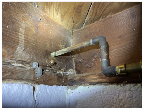
Some minor rot and signs of moisture on floor framing at back right in basement
