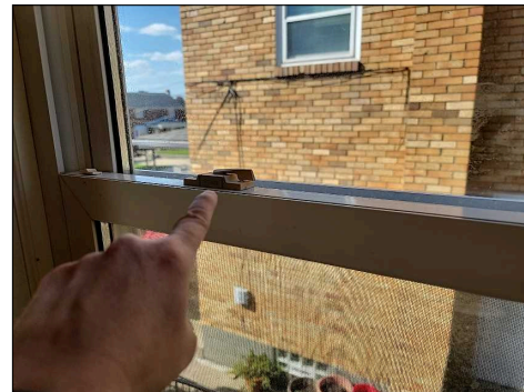
Window sashes would not line up to lock
