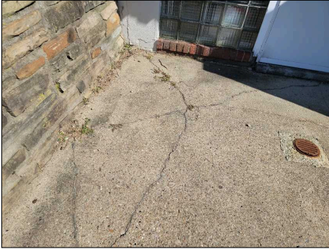
Various cracks to the concrete driveway
