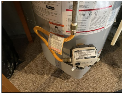
No drip leg on gas line to water heater
