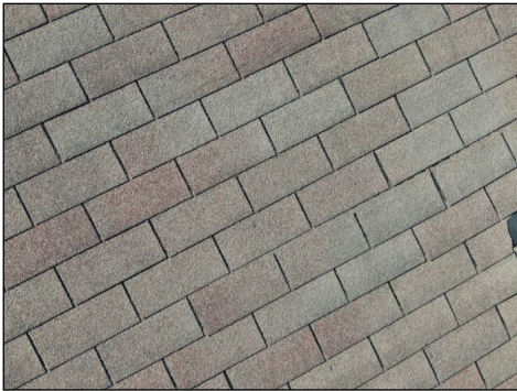
Granule loss and cracks to the roof
