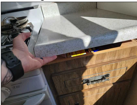
Kitchen countertop was not secured to the cabinetry
