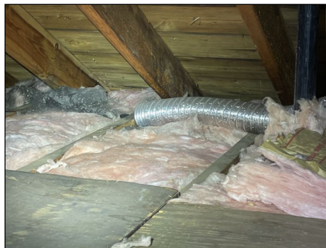
Bathroom vent fan discharging into attic
