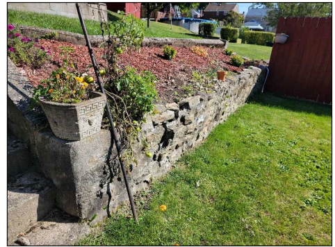
Bulging / leaning retaining wall at the back
