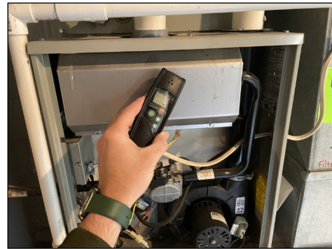
Furnace checked with a CO detector
