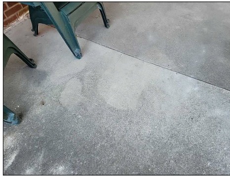
Cracks to the concrete slab observed at the back patio area
