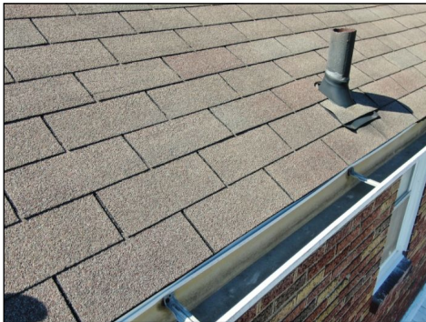
No drip edge flashing observed
