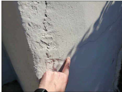
Cracks to the parge coat at the front
