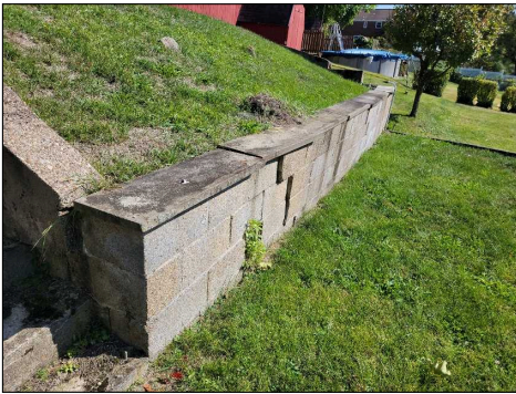
Cracked retaining walls at the rear
